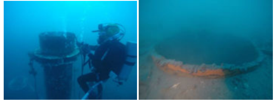
Decommissioning of pipeline
