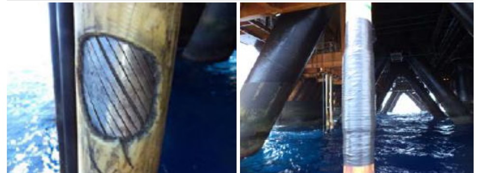
Risers and pipeline integrity
